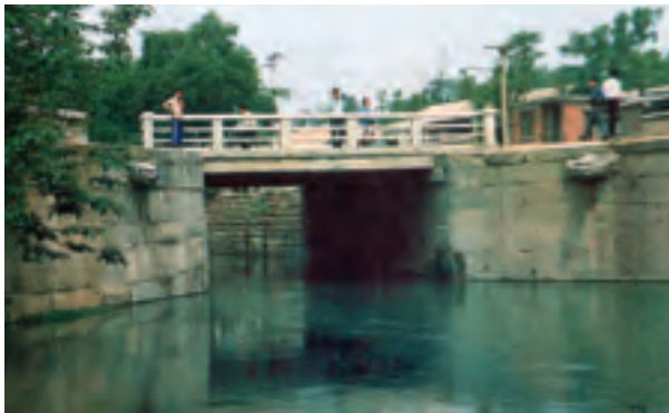
Guangyuan Water-Gate site: one of the twenty-four water-gates on Tonghui Canal
