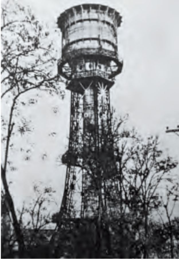
Water tower of the tap water works outside Dongzhi Gate
